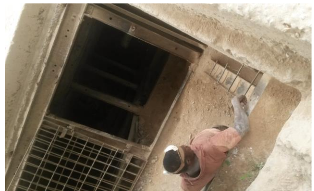
Fig. 4 Old Abandoned Adit with Metallic Support
