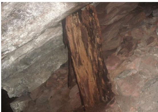
Fig. 13 Timber Support
